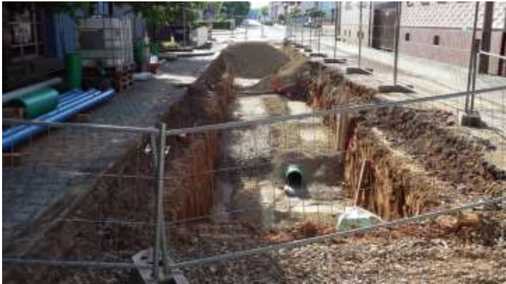
Example of “open cut” system
